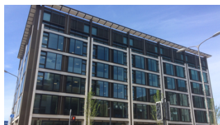
International Finance Centre, Jersey, UK
