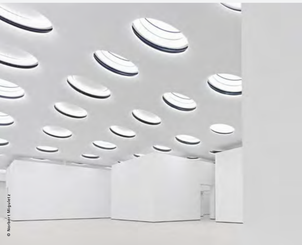
Städel Museum, Frankfurt am Main, Germany. The central design element in this concept created by Frankfurt-based architect's office Schneider + Schumacher are 195 ground-level skylights, double-covered with SEFAR® Architecture IA-80-CL, which ingeniously pick out the topography of the garden.
