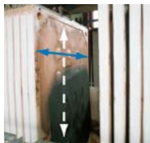
Application of SHT having high-strength warp (white) and elastic weft (blue)
